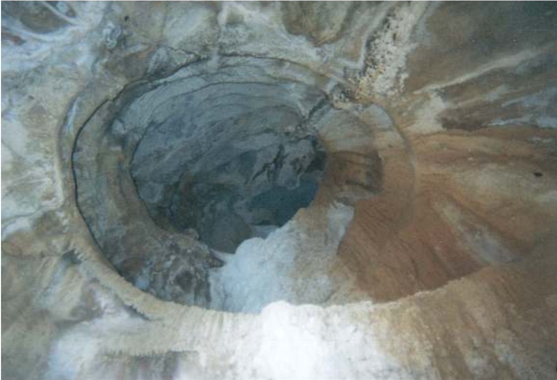
Ceiling detail in small dome near the Changing Room 11-12-06
